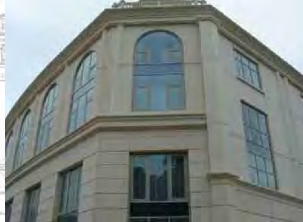
HOTEL RITZ - CARLTON POWERSCOURT COUNTRY WICKLOW - DUBLIN - IRLANDA JOHN SISK & SON LIMITED ARQº.: JAMES TOOMEY ARCHITECTS
